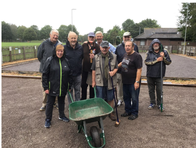
The hardy crew laying the grit on new terrain
